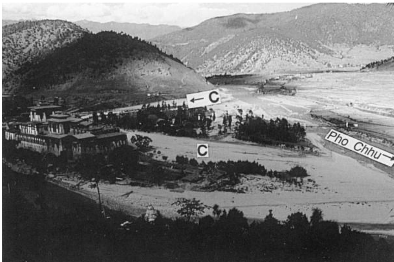
Figure 2. Flood damage in and around Punakha dzong due to Lugge Tso GLOF (6 & 7 October 1994), sourced from Watanbe & Rothacher (1996)
