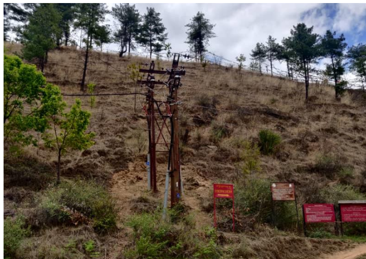
Plate 4. Transformers cause fire
