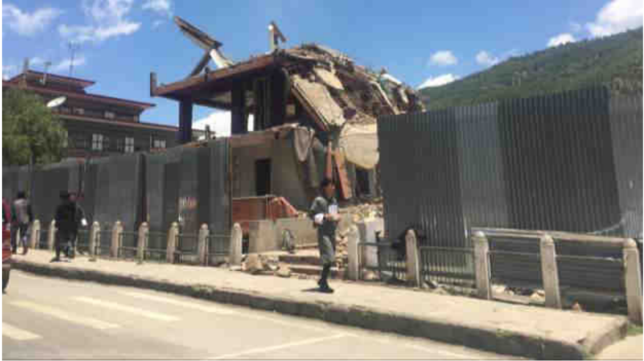
Figure 2-13 Demolishment of an old building in Thimphu
